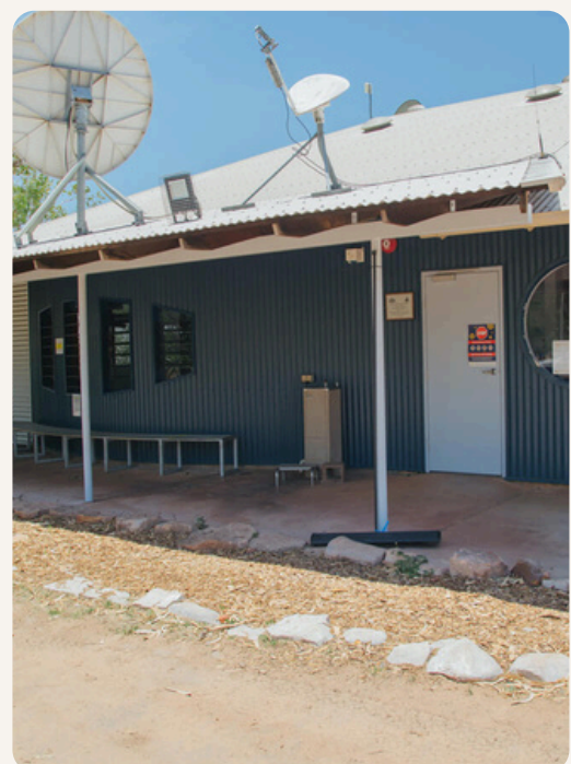
Image of Timber Creek clinic (supplied by KWHB website).
